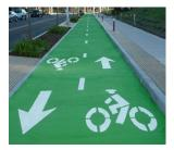
To designate a road or cycle track area as being for bicyclists, sometimes the pavement is of a different color. One option is to put a pigment into the pavement, as in the red pavement in the Netherlands. Another option is to paint the surface of the asphalt but this can wear off or be slippery. A new option is the product by Transpo Industries. The material is applied to the surface of the asphalt and comes in a variety of colors.
